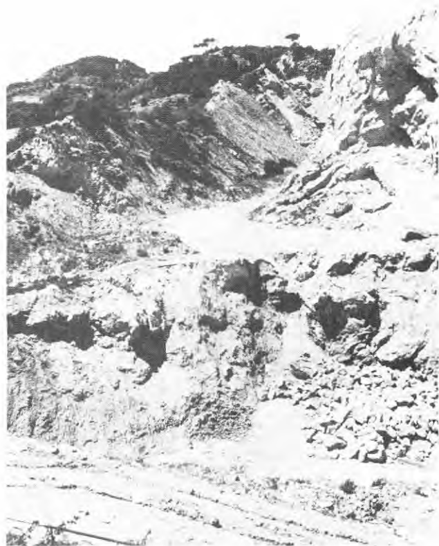
Fig. 1 – Western part of Monticino gypsum quarry in 1987. Old and new quarry floor are shown. Notice a steep dipping gypsum bedding plane in the upper half. Notice, by contrast, the chaotic setting of the lower quarry wall.
