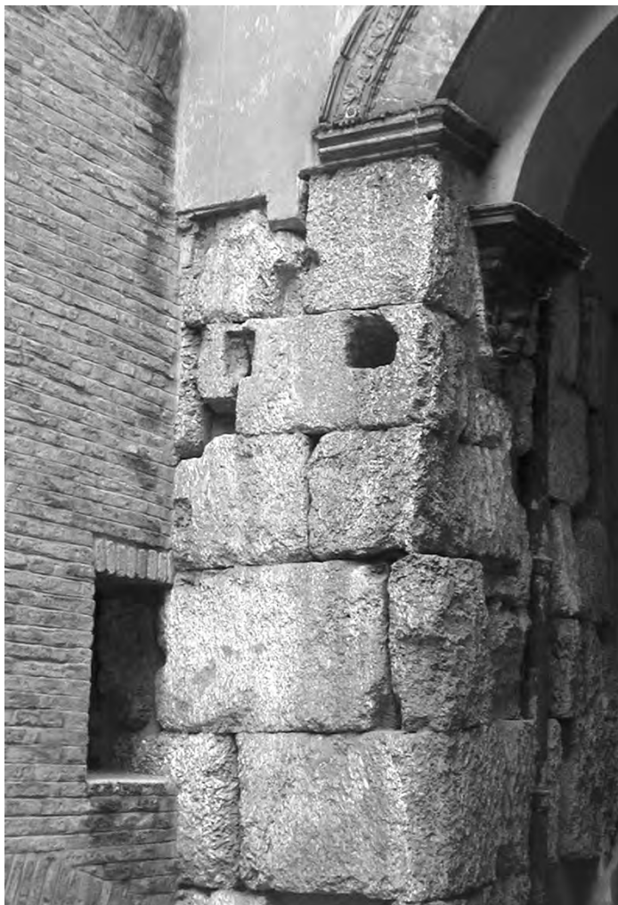
Fig. 1 - Remnants of the IV-VIII century AD selenite walls, preserved and recycled in the Ghisilardi Fava Palace at Bologna
